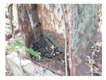
8. All structural members of the tower have corrosion. The extent of the corrosion varies. The bottom of the tower legs are the worst with complete loss of section in some members. The higher up members on the tower are not as severely corroded as the base. The corrosion condition lessens with mostly pitting and surface rust.
