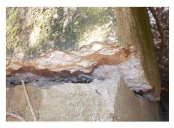
5. The foundation at Leg C has a much smaller crack and has also shifted. The crack continues completely through the pier. It is roughly 1/8" wide and occurs approximately 12"-14" below the base plate. The portion of foundation above the crack has shifted approximately 1/4" relative to the bottom portion in the direction of Leg D.
